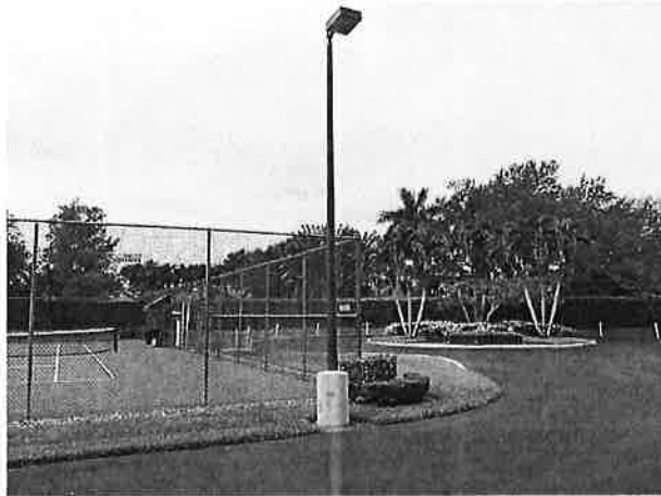
Light pole and fixture
