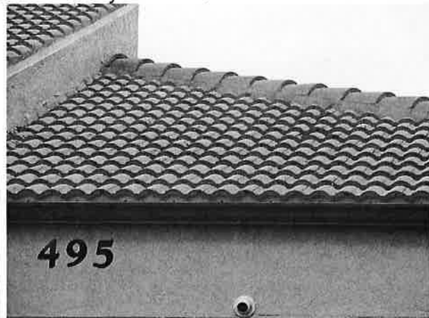
Concrete tile roof
