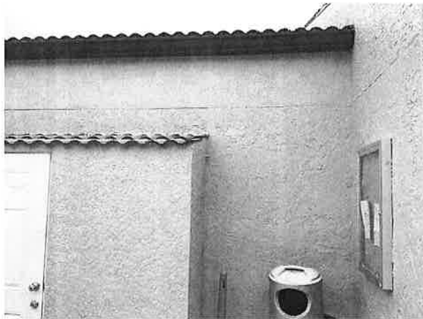
Stucco wall finishes
