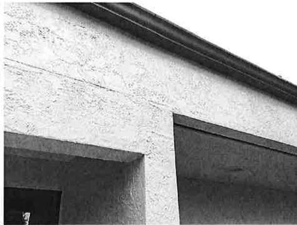
Stucco wall finishes
