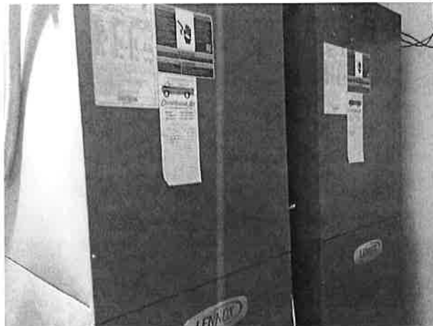
Split system air handling unit
