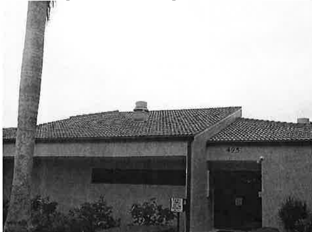
Clubhouse roof overview
