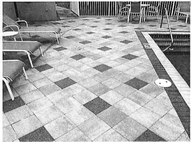
Paver pool deck overview
