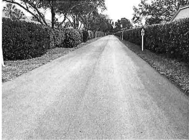
Asphalt pavement parking lot overview
