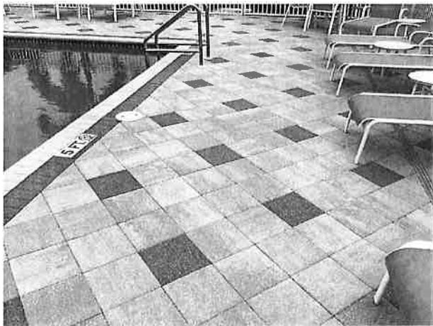
Paver pool deck overview
