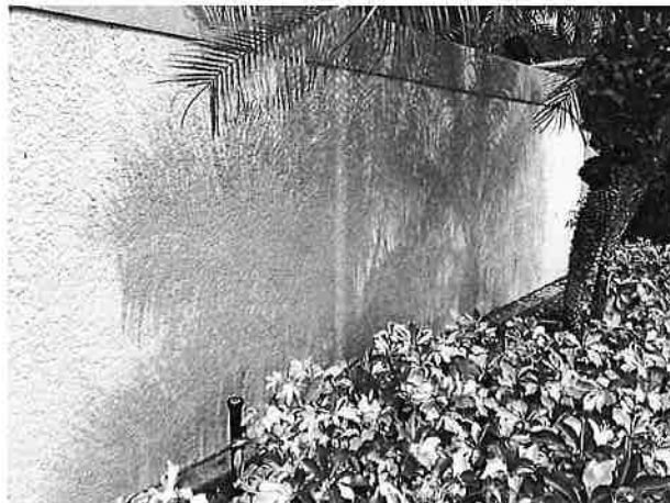
Stucco paint finishes
