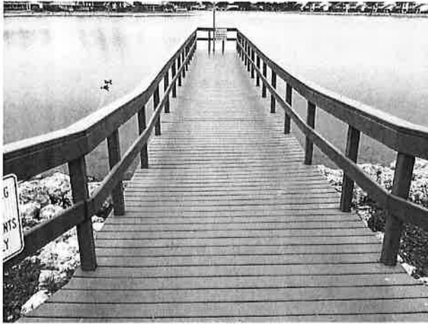
Dock with composite decking
