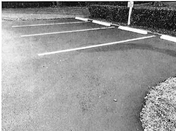
Asphalt pavement parking lot overview
