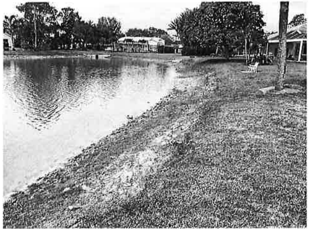
Minor shoreline erosion
