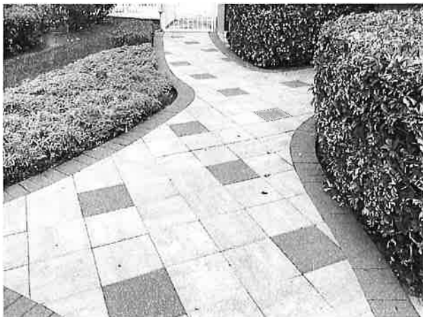
Paver pool deck overview
