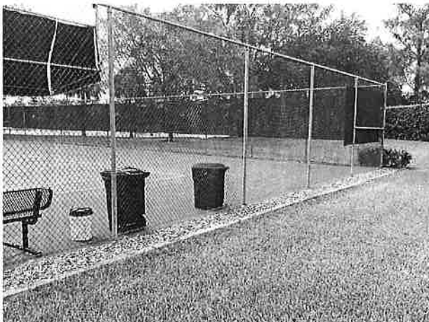
Chain link fence
