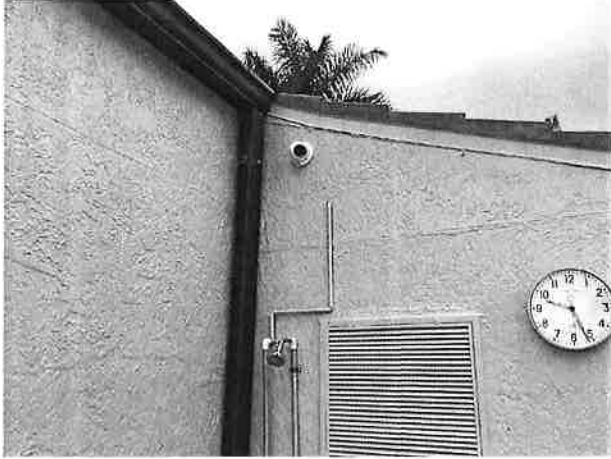
Security system camera
