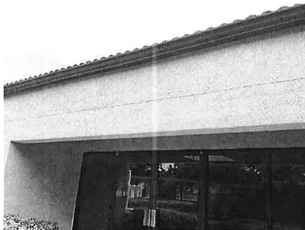
Stucco wall finishes
