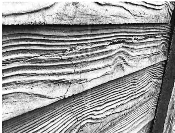
Concrete cracks
