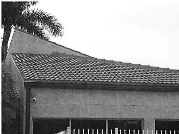
Concrete tile roof
