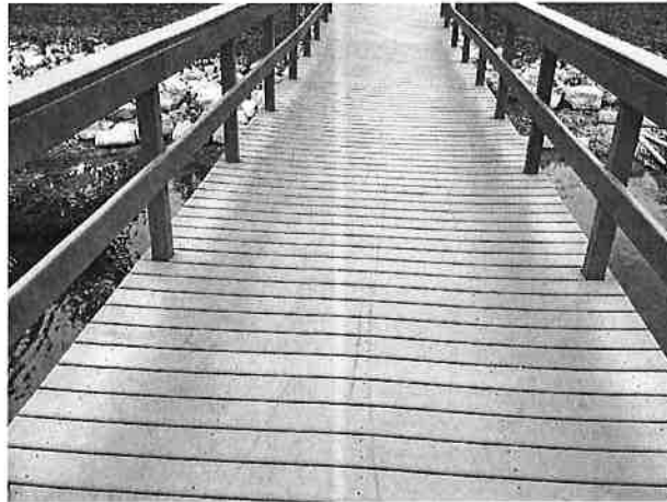
Dock with composite decking
