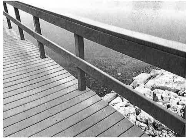
Dock with composite decking
