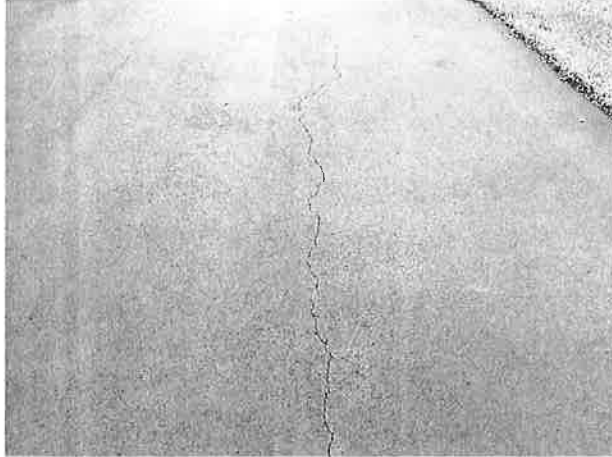
Pavement cracks
